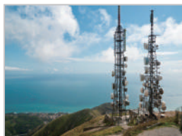
Telecom Backup Power
