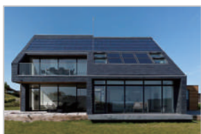
Off-grid Solar ESS
